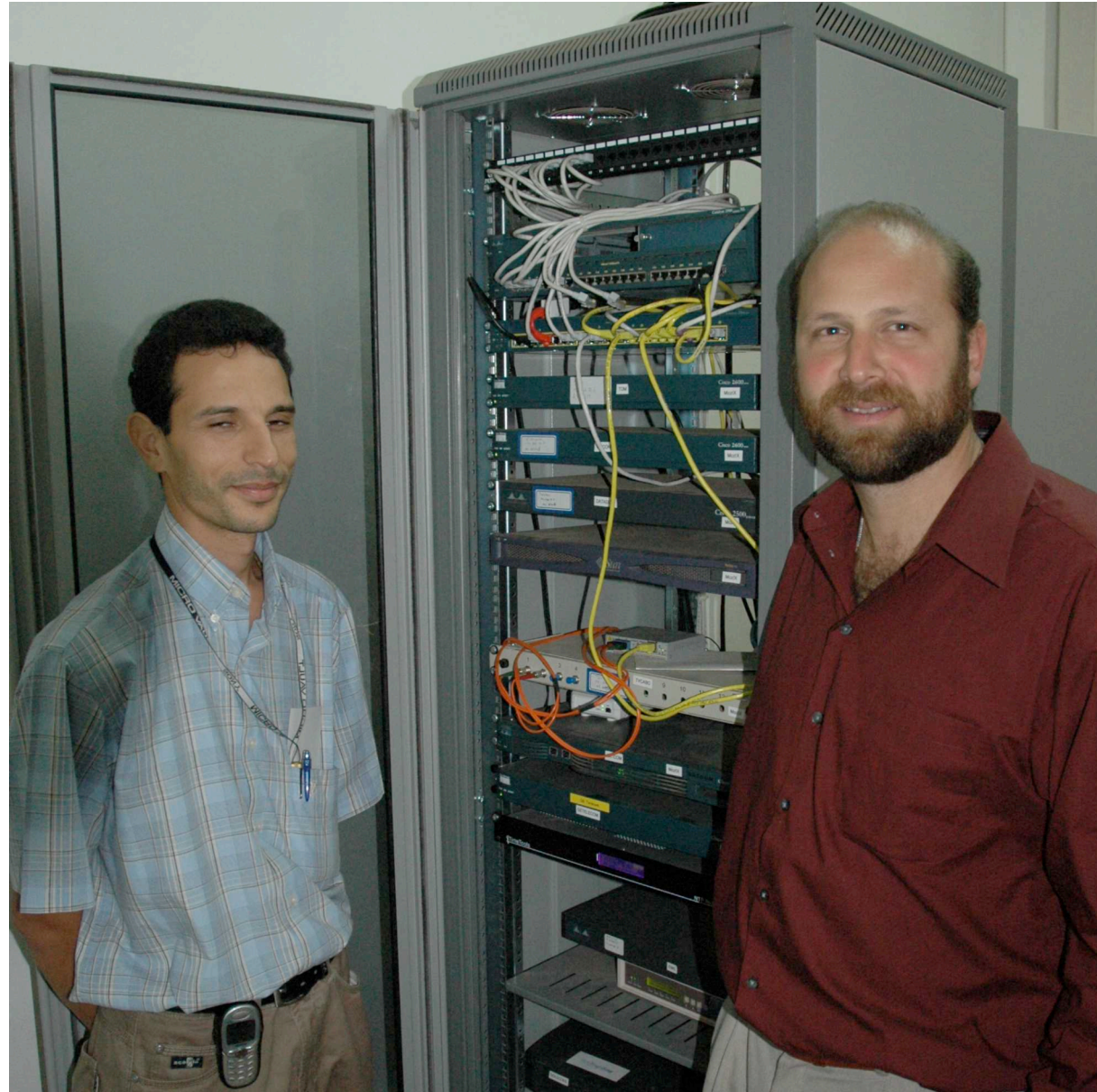
Mozambique Internet Exchange, Maputo
